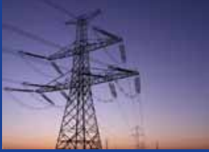
Power stations and power lines
